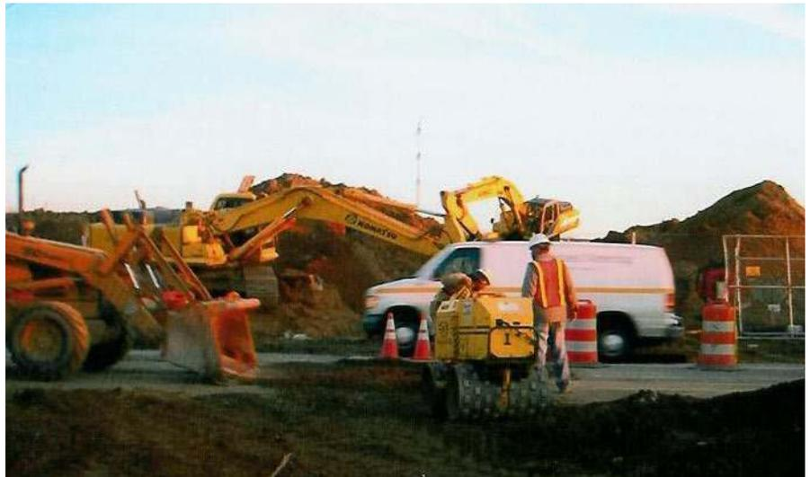
Eric Smith's company, Bond Construction was contracted to perform the following tasks: Install 3 facility sanitary sewer lines at an average 21 foot depth. Tied into 2 manholes across Lindbergh Blvd (State Highway & Septa Bus route). Tied into the city sewer main on the same line in one location across Lindbergh Blvd. Provided necessary traffic control, street restoration and paving to city specifications.
