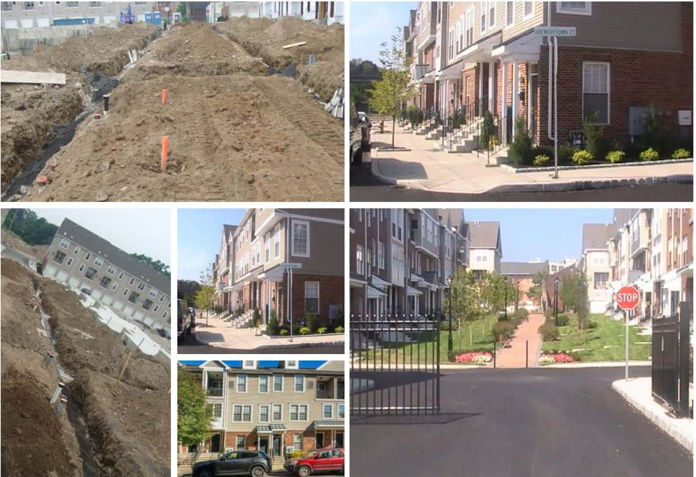
Eric Smith's company, Bond Construction was contracted to perform the following tasks: Excavation, backfill and installation of foundations and slabs for 144 houses. Concrete installation of all driveways, site and city curbs, site and city sidewalks and retaining walls. Installed all dry utilities (gas, electric, and communications). Installed site paving (base course).
