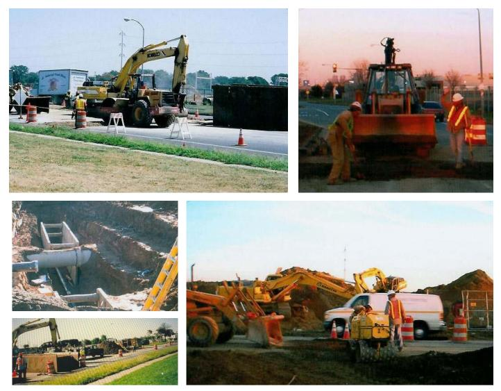
Eric Smith's company, Bond Construction was contracted to perform the following tasks: Install 3 facility sanitary sewer lines at an average 21 foot depth. Tied into 2 manholes across Lindbergh Blvd (State Highway & Septa Bus route). Tied into the city sewer main on the same line in one location across Lindbergh Blvd. Provided necessary traffic control, street restoration and paving to city specifications.
