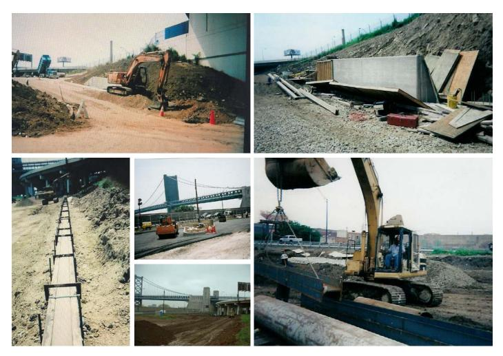
Eric Smith's company was contracted to perform the following tasks: Earthwork, retaining walls, storm sewer, sanitary sewer, domestic water, curbs, sidewalks and paving.
